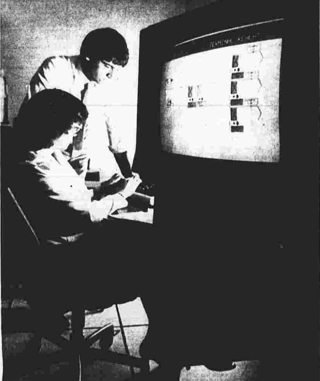
Technicians can monitor and control the heating, cooling and ventilating systems in a building complex with a building-management system developed in Farmington by United Technologies Building Systems Co. All data appears in a four-color diagram on the computer screen.
